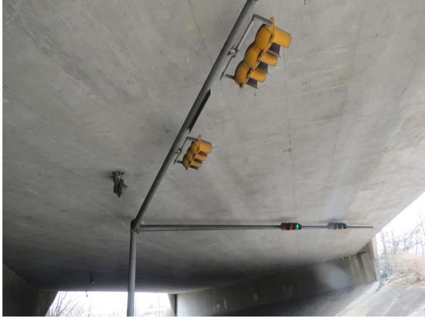
UNDERSIDE VIEW OF H.B.G.
