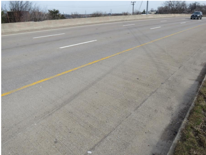
VIEW ACROSS TOP OF WEARING SURFACE WBL
