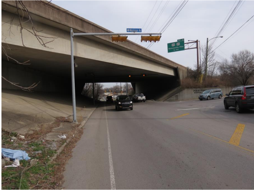
CLEARANCE VIEW RT. SIDE
