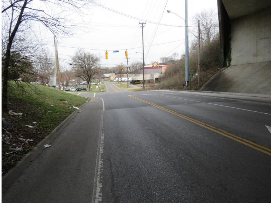
VIEW LOOKING NORTH ON BRANSFORD AVE.
